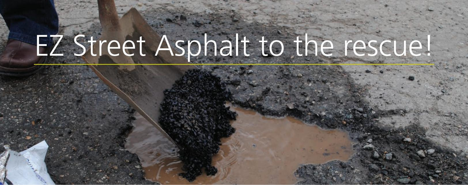
EZ Street is a high performance, polymer modified asphalt designed and produced with benefits exceeding that of regular asphalt but can be used with the same or better ease of cold mix.
